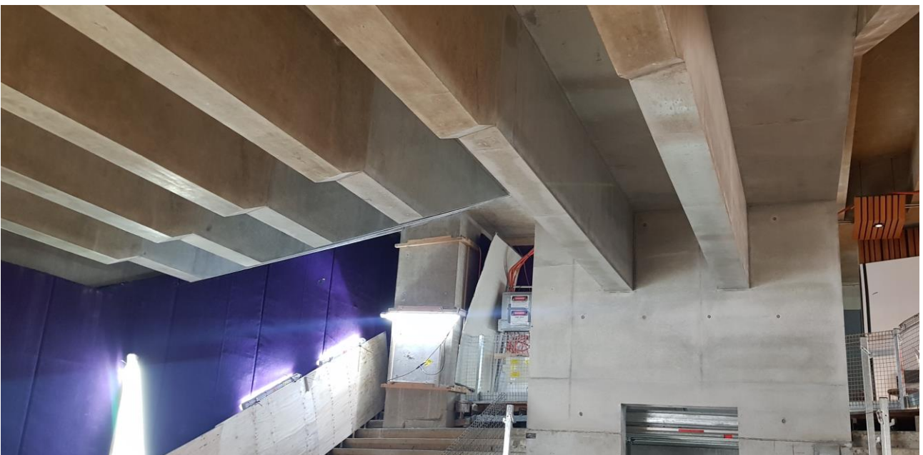
Photo 2: Concrete form between existing and new. Note change in colour.
