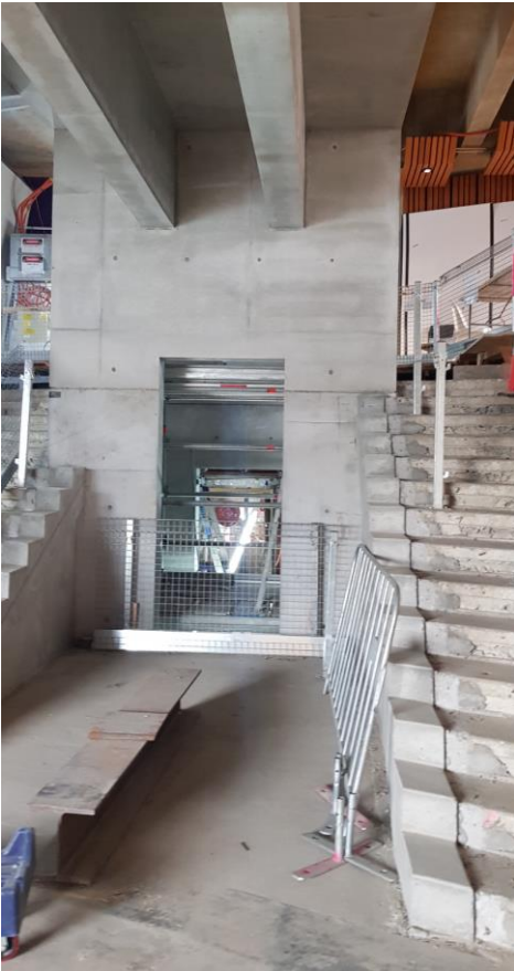
Photo 1: Main elevator shaft fully formed
