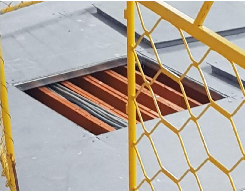
Photo 5: Services cut in
