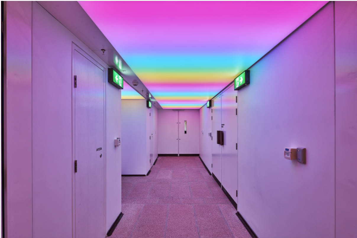
Plate 5: Completed Creative Learning Centre – Entry Passage
