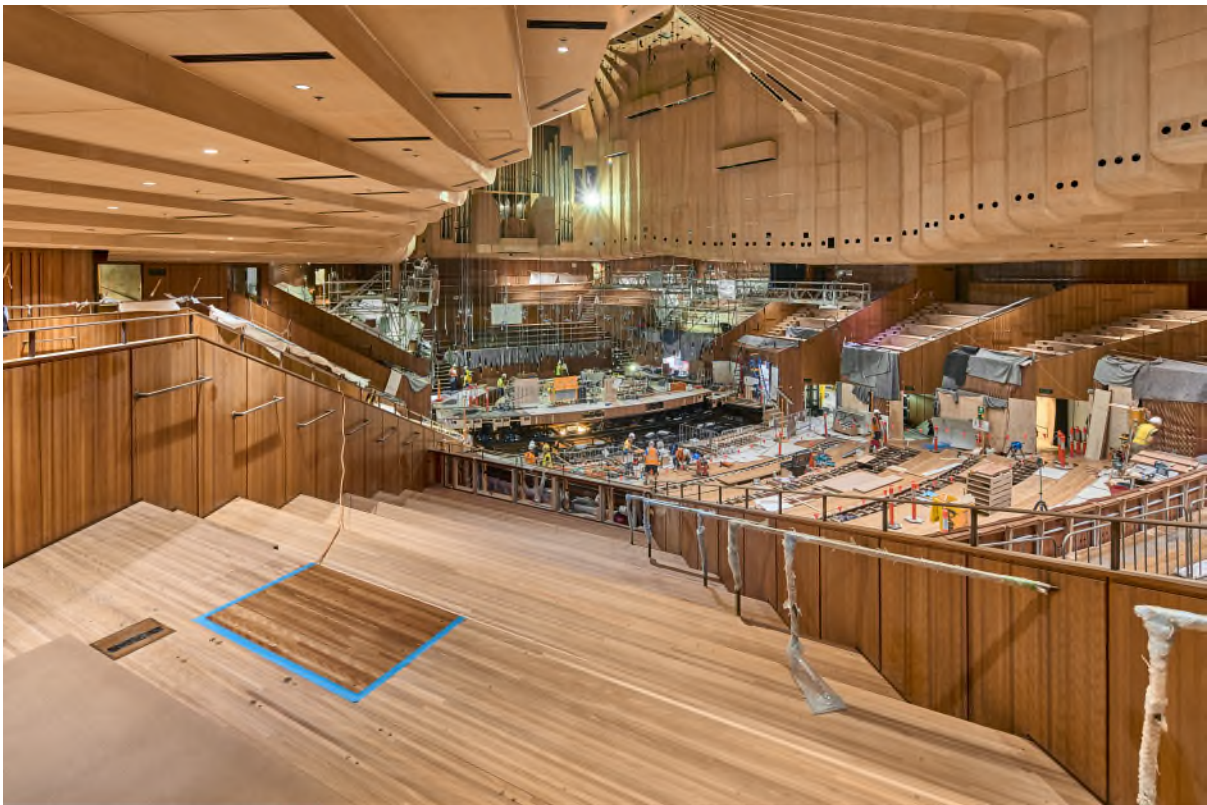
Plate 10: Concert Hall – View from Circle Box towards Stage
