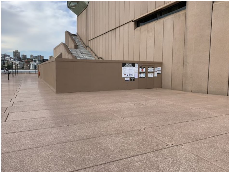
Plate 1: Main Site Entry (showing hoarding)
