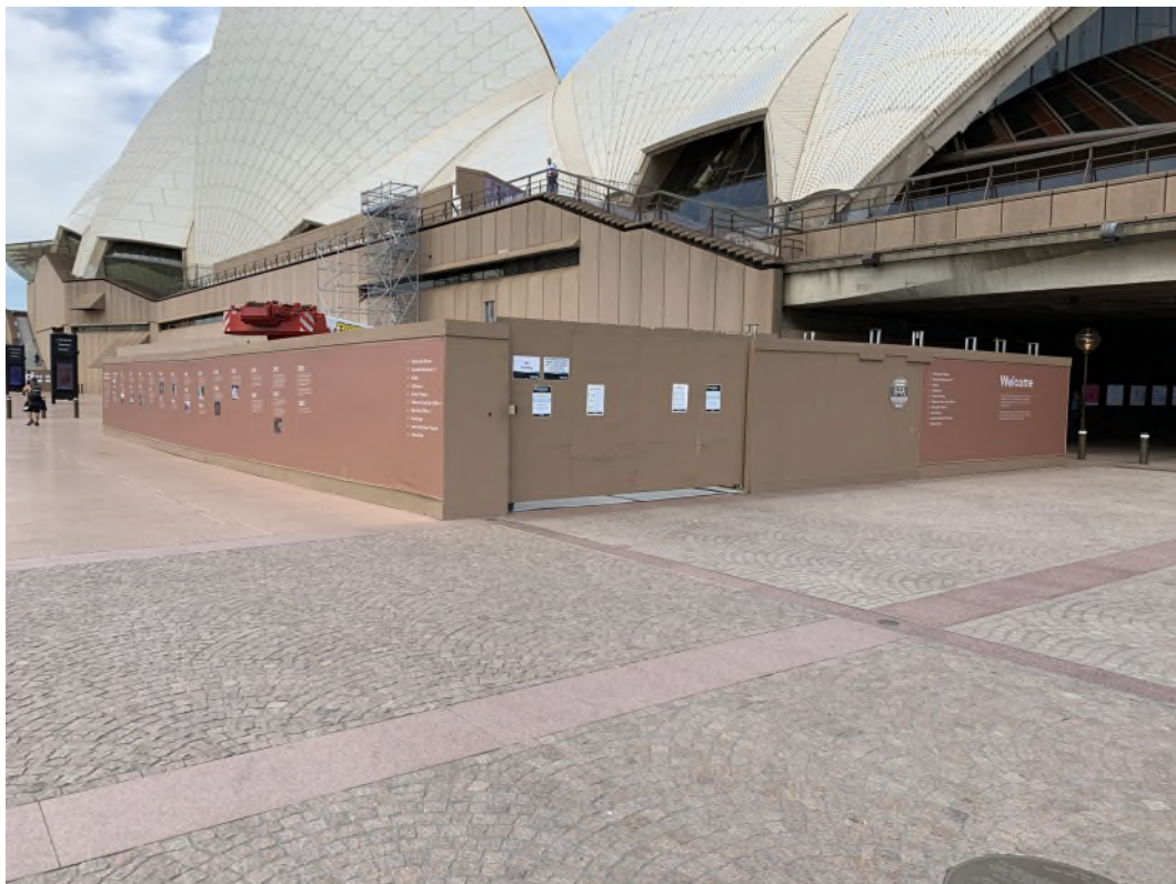
Plate 3: Hoarding around lifting zone, showing interpretation material
