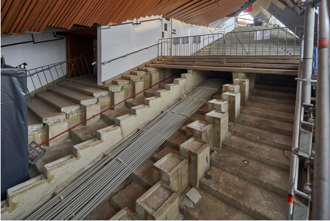
Plate 6: Eastern Foyer stair demolition for passageway May 2020
