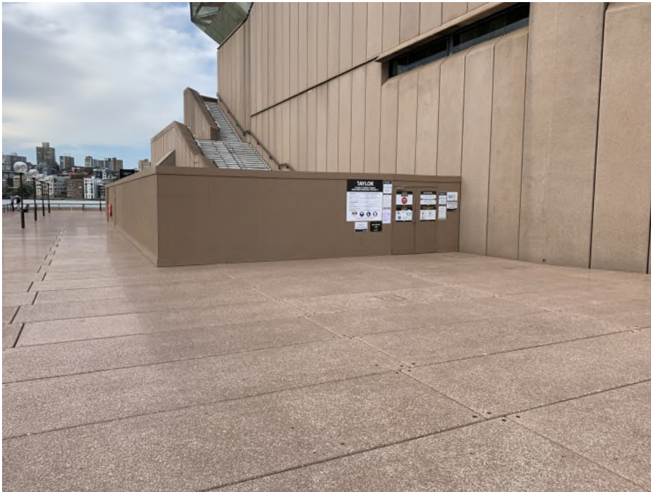
Plate 1: Main Site Entry (showing hoarding)
