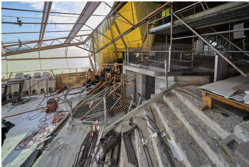
Plate 4: Concert Hall Construction of Lift 30 (18 February 2021)
