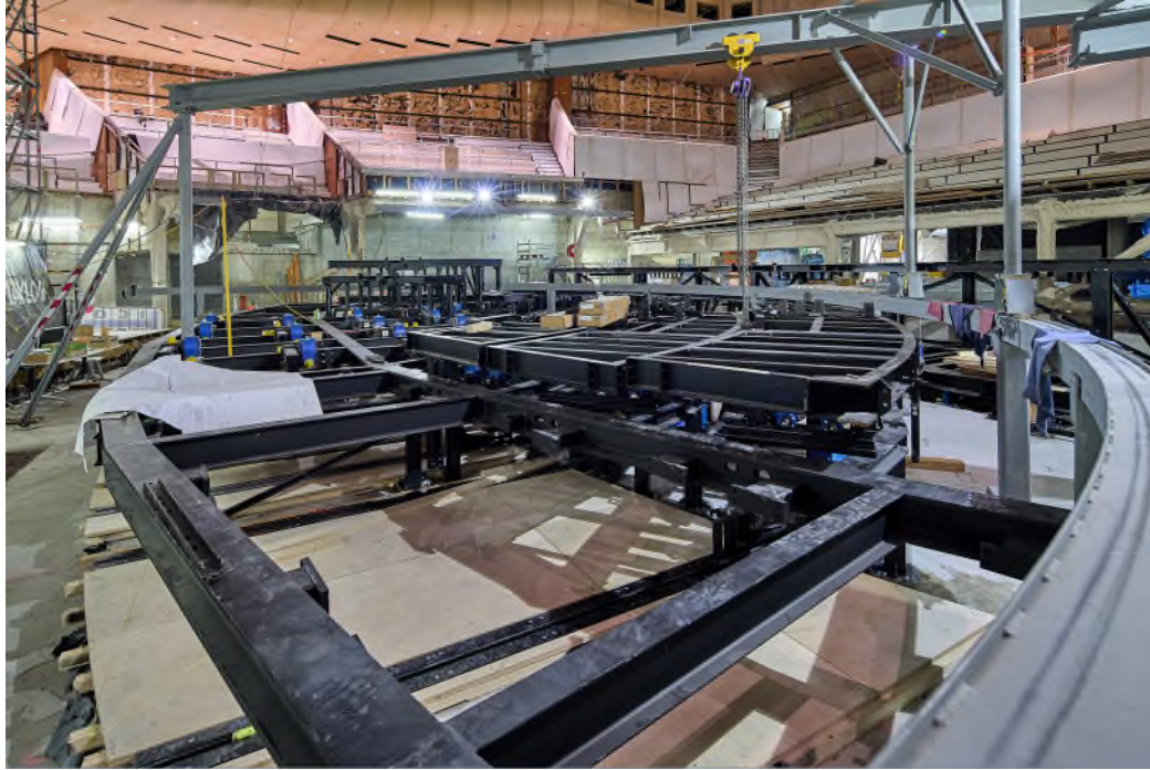
Plate 5: Installation of Concert Hall Stage Machinery (13 January 2021)
