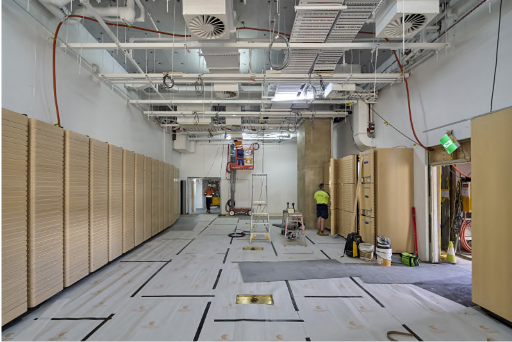
Plate 7: Internal Fitout of Creative Learning Centre (13 January 2021)
