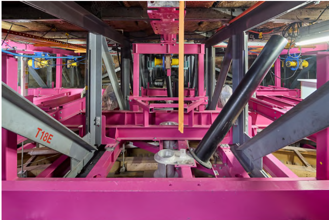
Plate 6: Strengthening of Structural Steel Members in Concert Hall Ceiling (13 January 2021)
