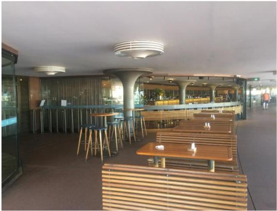
Figure 7: Lower Concourse mushroom columns and louvered disc light fittings (Source: Keylan)
