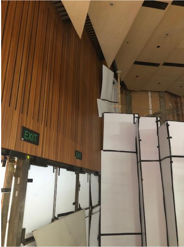
Photo 14: Heritage listed wall panelling
