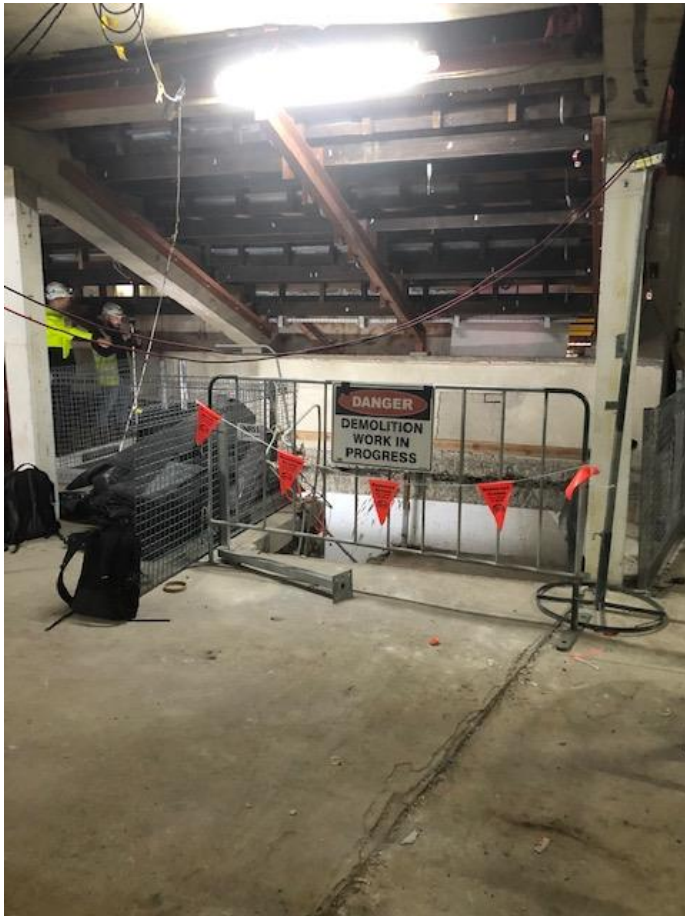
Photo 12: Demolition work in progress in the roof above the Concert Hall
