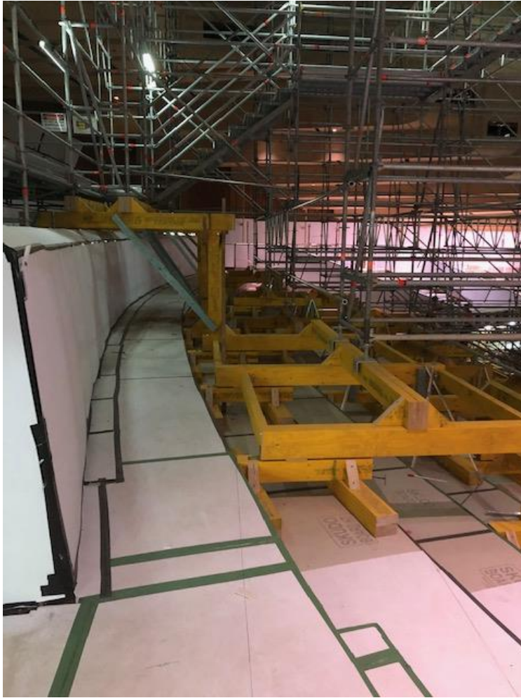
Photo 6: Concert hall refurbishment works
