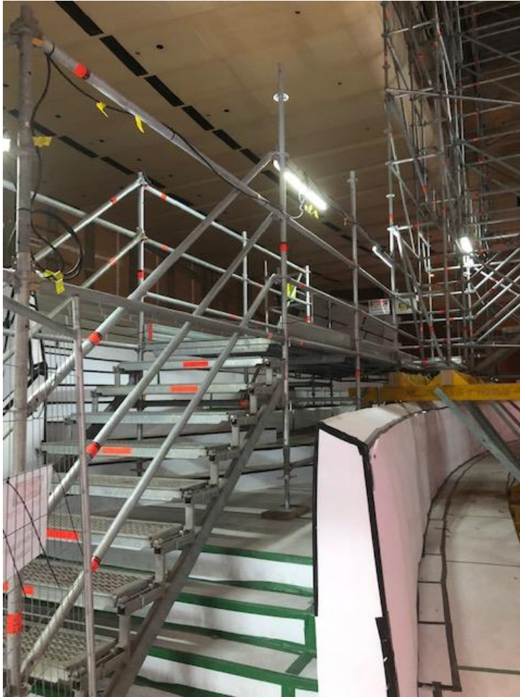
Photo 5: Concert hall refurbishment works in progress
