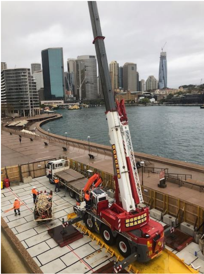
Photo 10: Crane in Taylor site compound 2
