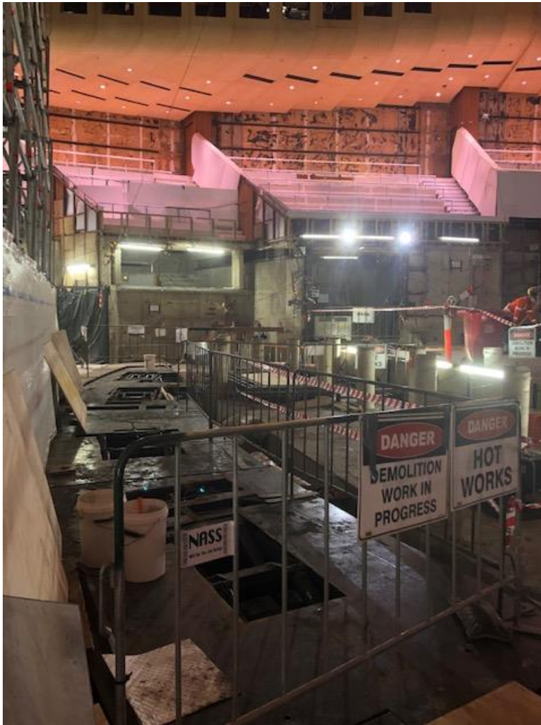
Photo 7: Concert Hall works
