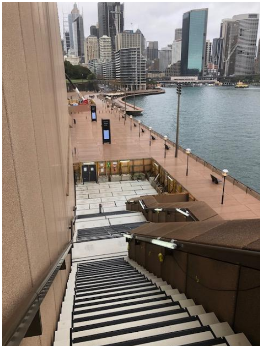
Photo 21: Taylor external compound looking south
