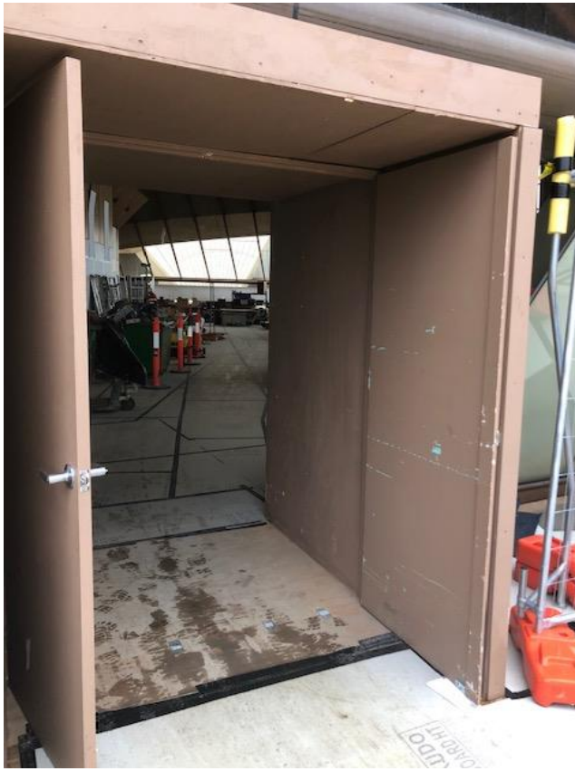
Photo 13: External temporary timber door to the Concert Hall (upper level)
