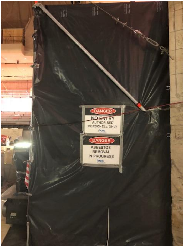
Photo 2: Asbestos Removal Works- Concert Hall
