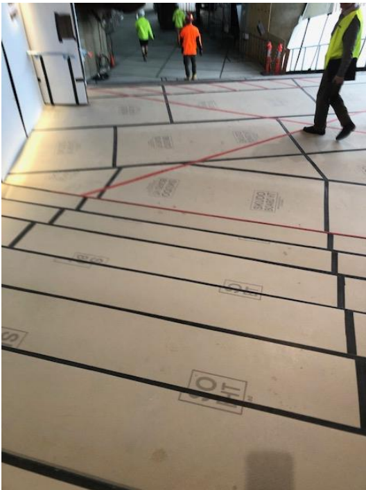
Photo 18: Protection to heritage flooring and stairs
