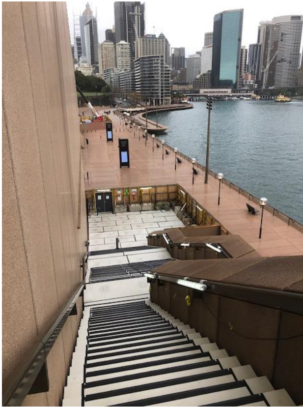
Photo 22: Taylor external compound looking south 2
