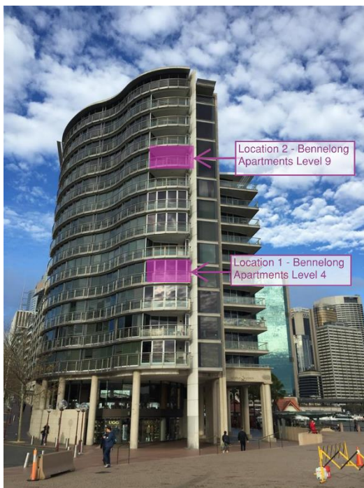
Figure 2: Noise monitoring location at Bennelong Apartments (left)
