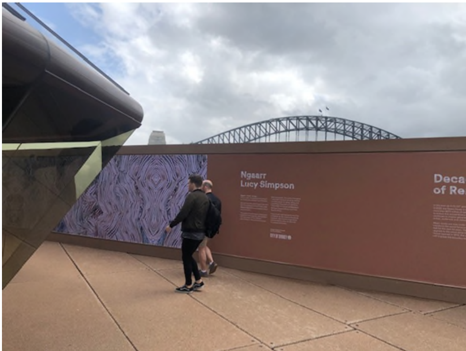
Construction hoarding on podium
