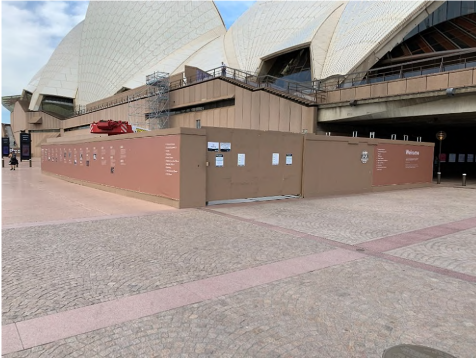
Construction hoarding around crane compound – heritage interpretation material along hoarding on Western Broadwalk
