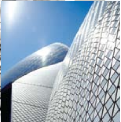
Utzon spent three years developing the ceramic tiles – there are over one million tiles of 17 different varieties in gloss matt, white and cream finishes. Utzon wanted the shells to contrast with the dark water under the deep blue Australian sky – like clouds or sails on the water.
