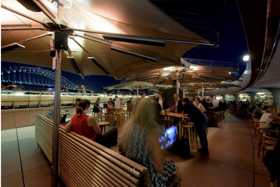
Figure 35: Underside of an existing umbrella indicating the effect of up-lighting on the membrane fabric which is used to generate a low glare ambient glow
