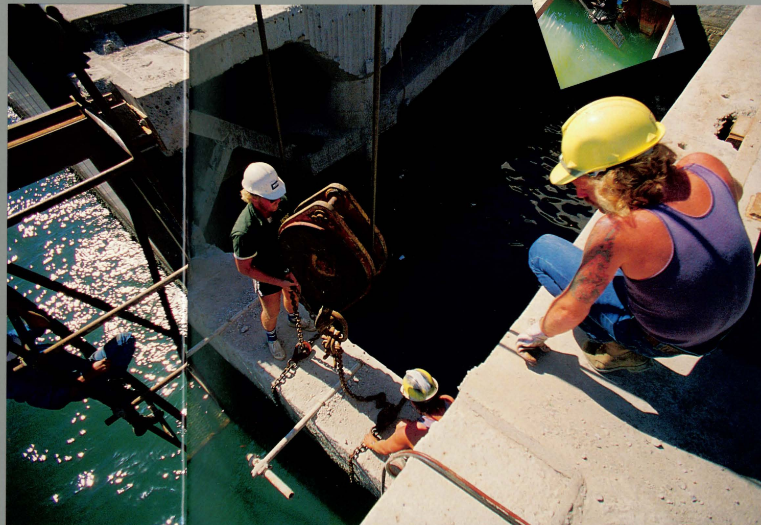
A diver goes down to excavate silt from the cofferdam.
