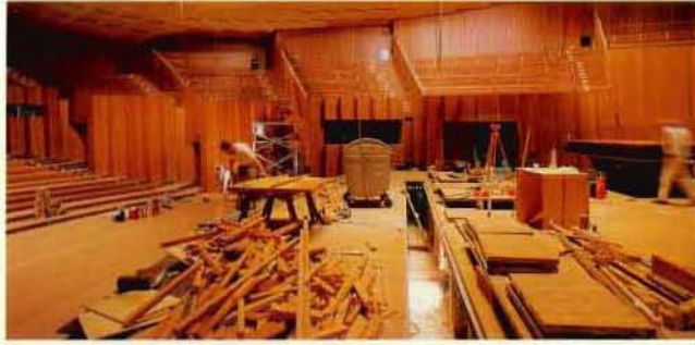
Renovating the Concert Hall stage
