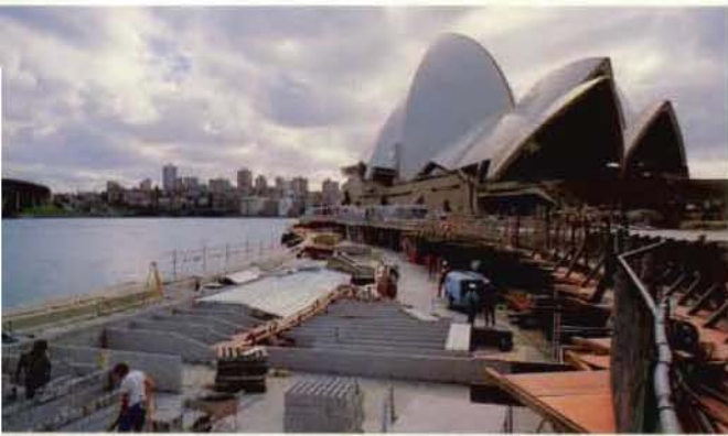
The lower concourse level takes shape
