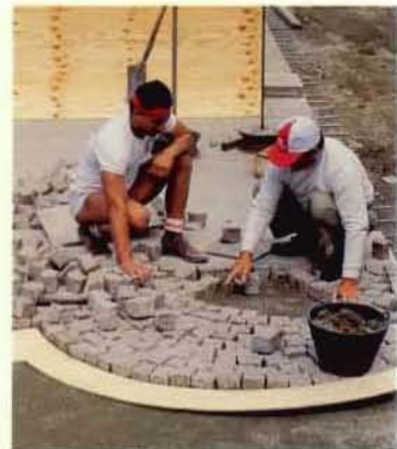
Laying the cobblestones
