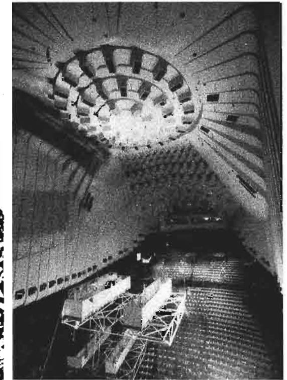
WORKING PLATFORM SUSPENDED FROM CONCERT HALL CEILING
