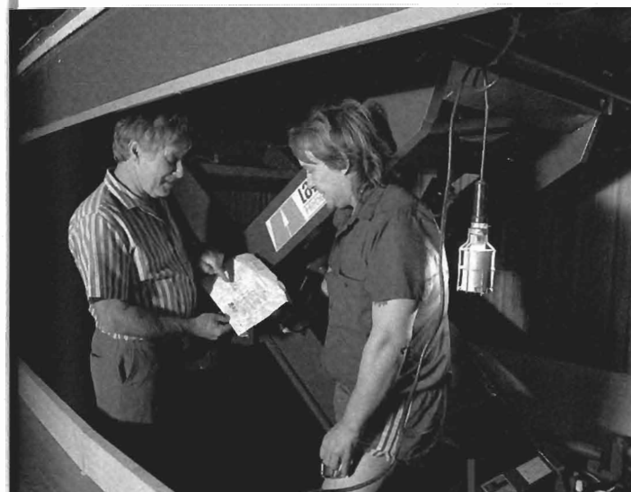
Checking the new Concert Hall stage extension
