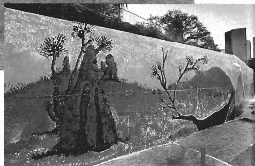
Decorating the temporary wall containing car park work on site
