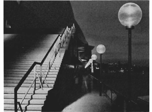
The lighting for the steps is placed under the hand rails. The circular acrylic lamps surround the House on the broadwalk. They have a concealed lamp which reflects from the top to give a lighting effect.
