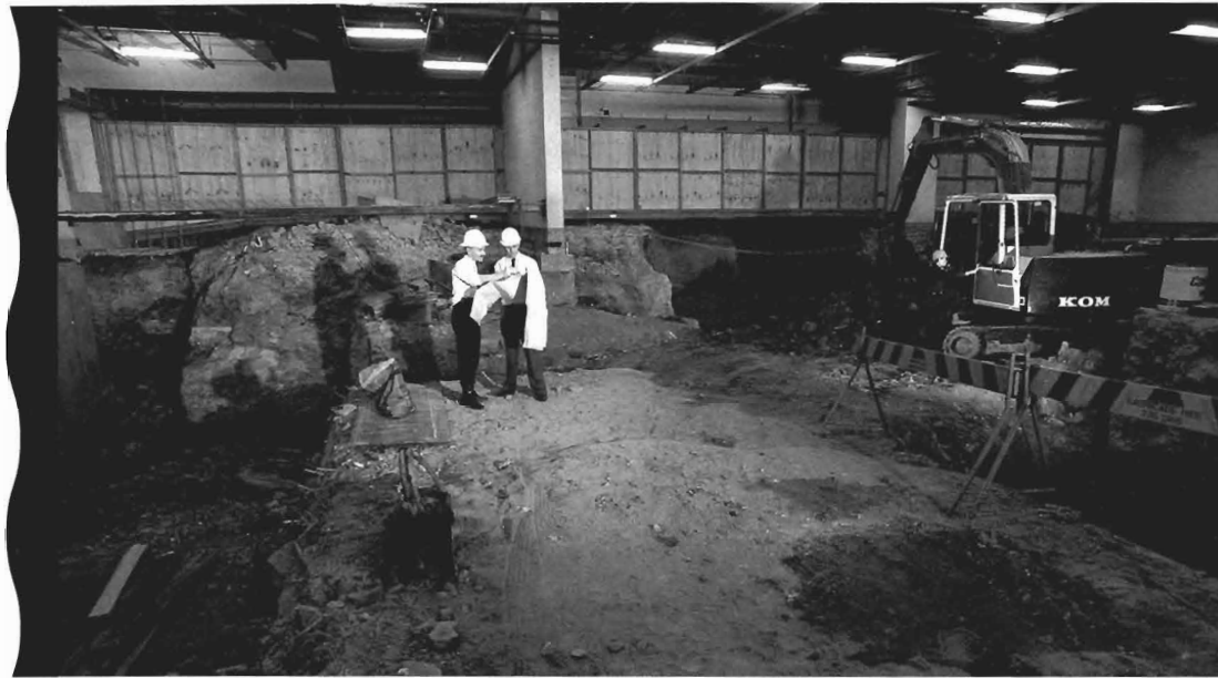
Excavation of floor area
