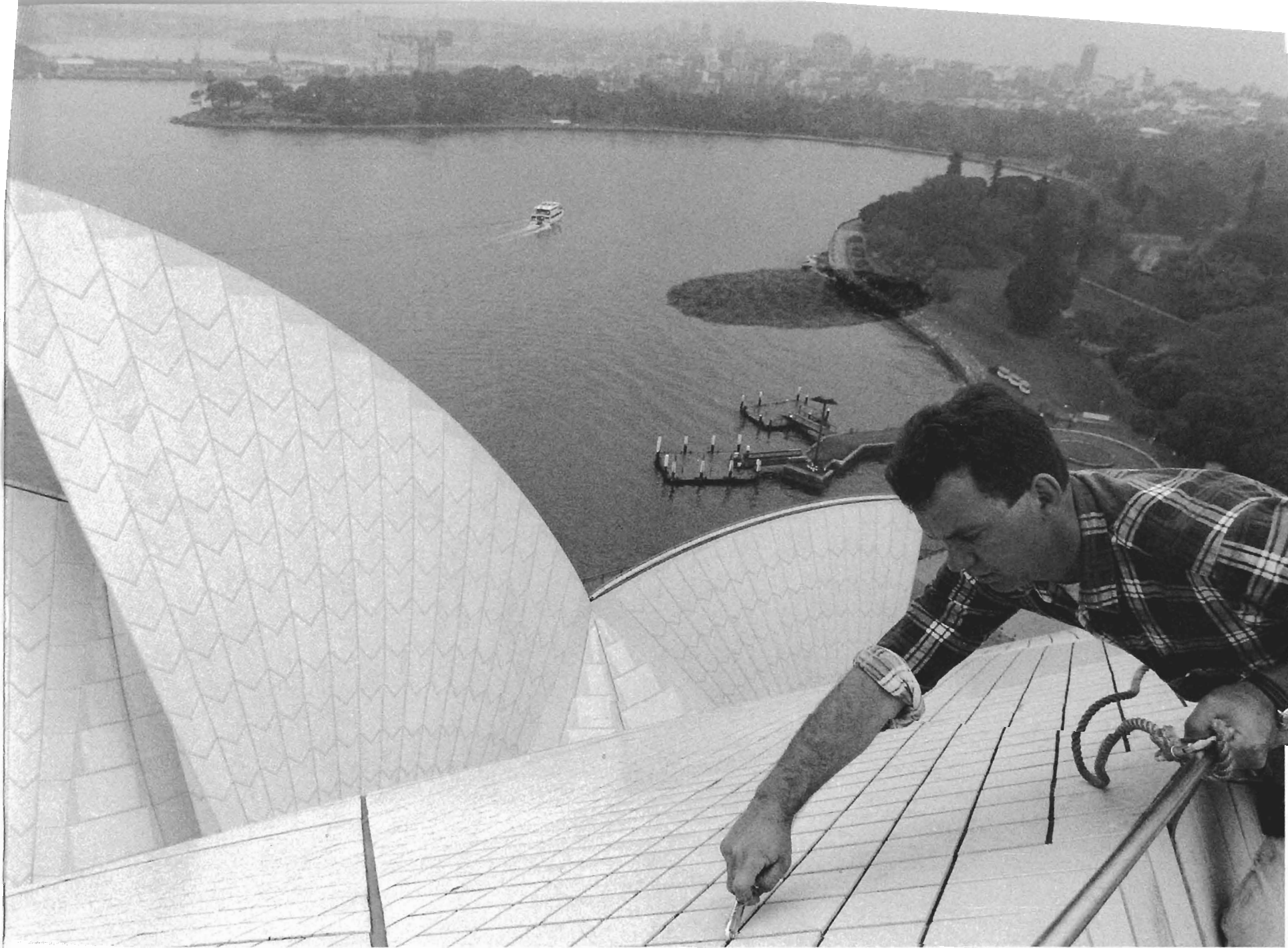
Resealing tiles Photograph Robert McFarlane
